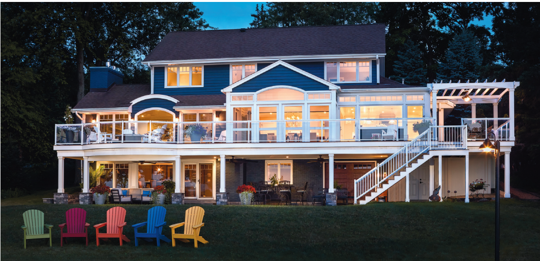
Bartelt. The Remodeling Resource earned an award in the whole house remodel category. While the homeowners loved the location of their lake home, it lacked character and didn't fit their lifestyle. The Bartelt team was asked to create a home that accommodated entertaining and took advantage of the lake views. After removing walls and reconfiguring the space, the first floor now features a wall of windows that runs the entire length of the home. The crisp blue and white exterior colors are a nautical nod to the home's lakeside location.
