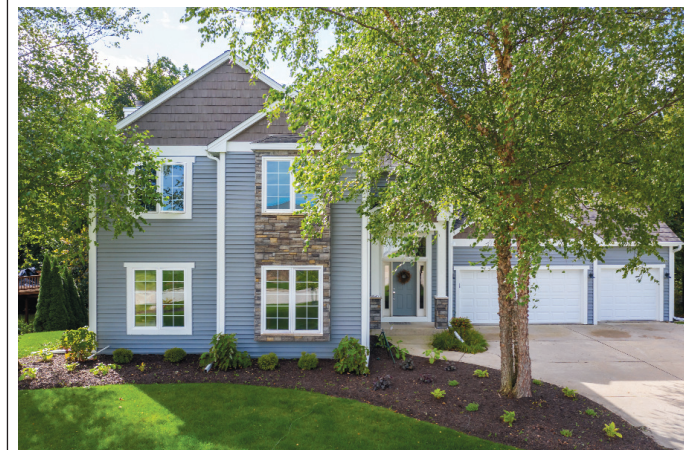
Project by Allrite Home & Remodeling, NARI Milwaukee Remodeler of the Year Residential Exterior Under $50,000 Gold Award Winner
